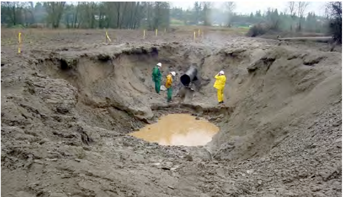
Failure of a natural gas transmission pipeline. In this incident there was no explosion or fire, the crater was created by the pressure of the gas coming out of the pipeline. Note how far the pipe in the upper right corner was thrown.
