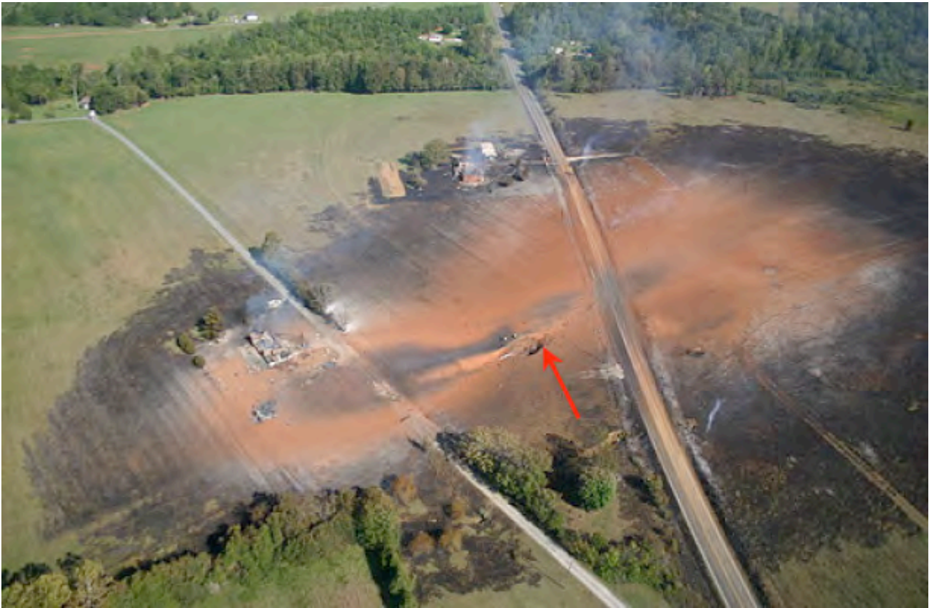
Failure of a natural gas transmission pipeline. Arrow shows point of failure. Note how far from point of failure houses were destroyed
