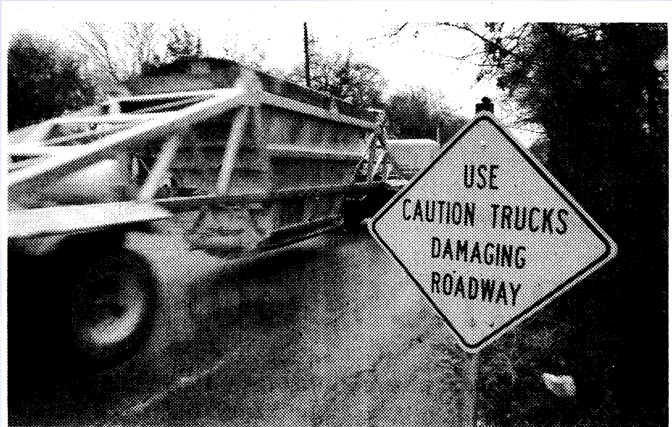
A sign warns drivers of road damage from heavy trucks on Farm Road 3325 in the Azle area.
